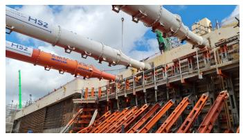
Altrad RMD Kwikform (Altrad RMDK) has supplied above and below ground temporary works to assist primary contractor Skanska, Costain and STRABAG (SCS) joint venture (JV) with the construction of HS2's West Ruislip Portal, demonstrating its engineering expertise to increase project productivity.
