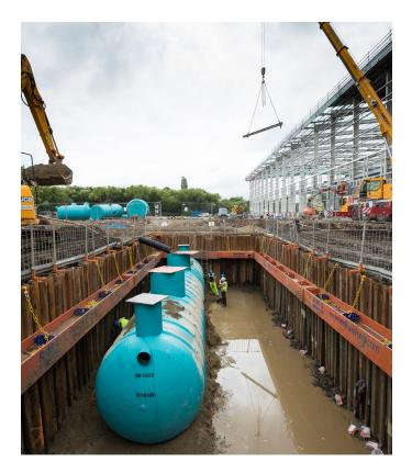
An underground waste food treatment facility has been constructed by groundworks and construction specialist Euro-City Eastern at SEGRO Park, Heathrow. Operations Director, Michael English, turned to RMD Kwikform to provide a safe and cost-effective groundshoring solution to build a temporary cofferdam in which to position two 70,000-litre grease trap tanks.
