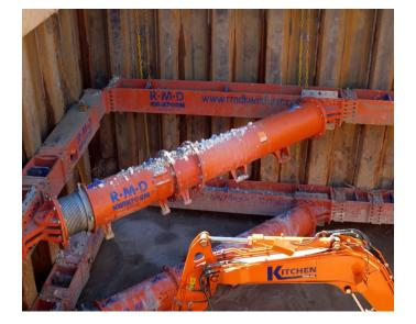
A key feature of the Tubeshor 610 prop, in addition to the Hydraulic lock off, is the mechanical lock off mechanism that carries the load.
