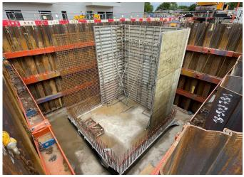
Temporary works specialist, Altrad RMD Kwikform (Altrad RMDK), recently provided K Rouse Civil Engineering a bespoke integrated ground shoring and formwork temporary works solution to support a challenging excavation for the construction of the new Fujifilm Borealis biotech manufacturing facility in Billingham.
