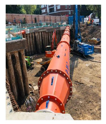
The angle between the prop and the capping beam is about 45° but varies both horizontally and vertically due to the geometry of the permanent works.
