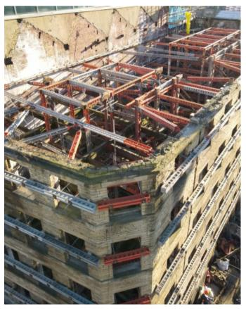
Altrad RMDK engineers specified a bespoke temporary works solution to successfully support the structure, using a mix of Megashor and Superslim soldiers to secure the walls to enable the contractors to progress with rebuilding Galem House floor by floor.
