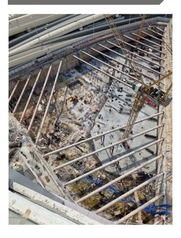
Altrad RMD Kwikform (Altrad RMDK) has supplied a ground shoring solution to support a challenging large-scale excavation in Abu Dhabi in the Middle East – one of the largest excavations in the company's history, featuring a maximum depth of 14.25m, and approximate volume 111,050 m3. The Tubeshor solution was chosen for its ease of use and installation, improving productivity on site while mitigating the risks posed by the challenging site environment.
