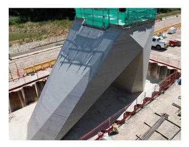
The analysis of the formwork was one of the most challenging ever undertaken by Altrad RMDK and pushed the boundaries of what is possible with conventional software. An elastic analysis was carried out on the complete structure and contained over 13,000 individual members.
