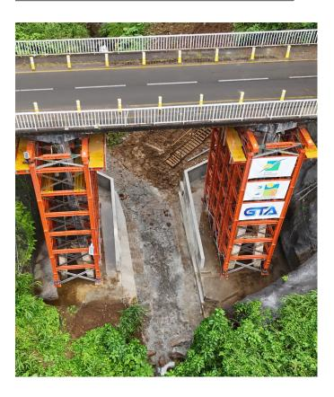
Temporary works specialist Altrad RMD Kwikform (Altrad RMDK), recently joined forces with sister company Altrad Coffrage & Etaiement to reinforce Pont des Ecrevisses, a bridge on the RN 3 in Saint-Claude, Guadeloupe. The reinforcement was necessary to reestablish the bridge's structural integrity after its piers were weakened by storm Fiona a few years ago.
