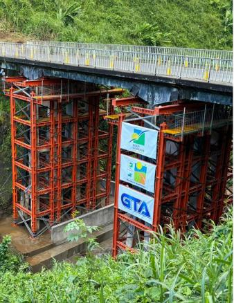
Altrad RMDK engineers suggested implementing a single flat concrete foundation. This approach not only avoided the risk of intensifying the damage, but also simplified the erection process by providing a stable base for the bridge components. The flat foundation ensured uniform support, allowing vehicles, loads and people to successfully navigate across the bridge.
