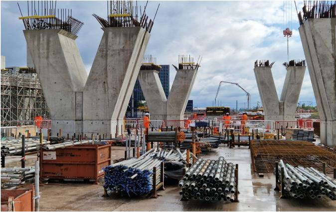
Altrad RMDK achieved the deck profile with a system of aluminium wallings & Superslim primary beams – which sat on the top of the falsework and incorporated a cantilevered support to the wings of the deck. Again, this ensured the structure was then all internally supported – mitigating the need for use of external props to the ground.
